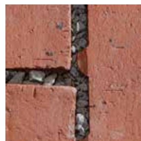
Joint drainant de 6 mm = part des joints: 10%
