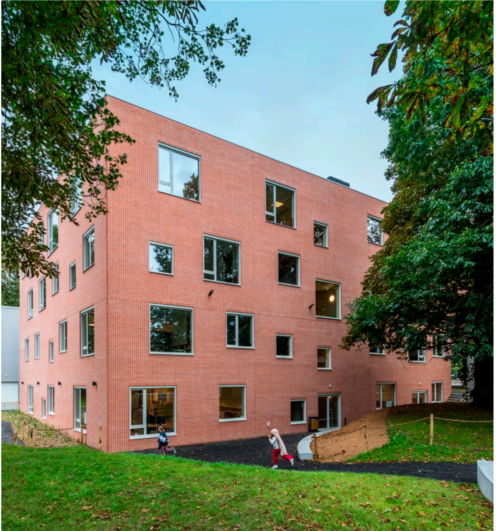
The use of a false joint creates a seemingly simple stacking of square bricks in the façade. Design: Oskar architecten, Dilbeek
