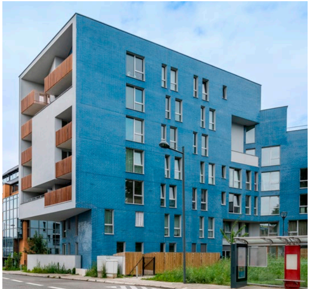
Pierre Blondel Architects finished the façades with a combination of blue glazed ceramic facing bricks and white plasterwork. The dual use of materials points to the interaction between the city and the urban periphery.
