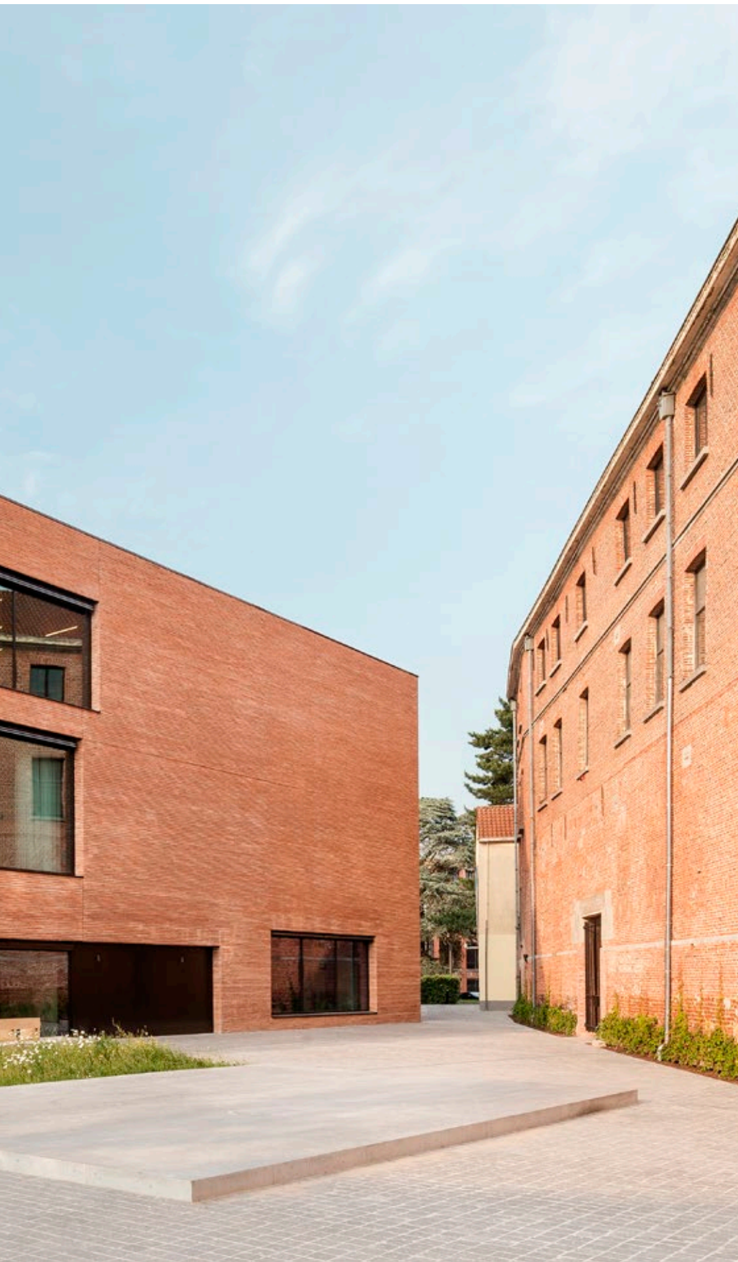
KAAN Architects (NL) chose long, narrow Waterstruck facing bricks for library Utopia in Aalst to elegantly integrate the 19th-century Pupil School while rejuvenating the urban landscape.
