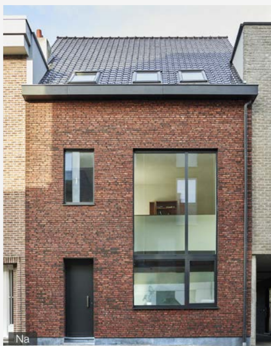
Renovatiecase Mechelen © ROVE Architecten
