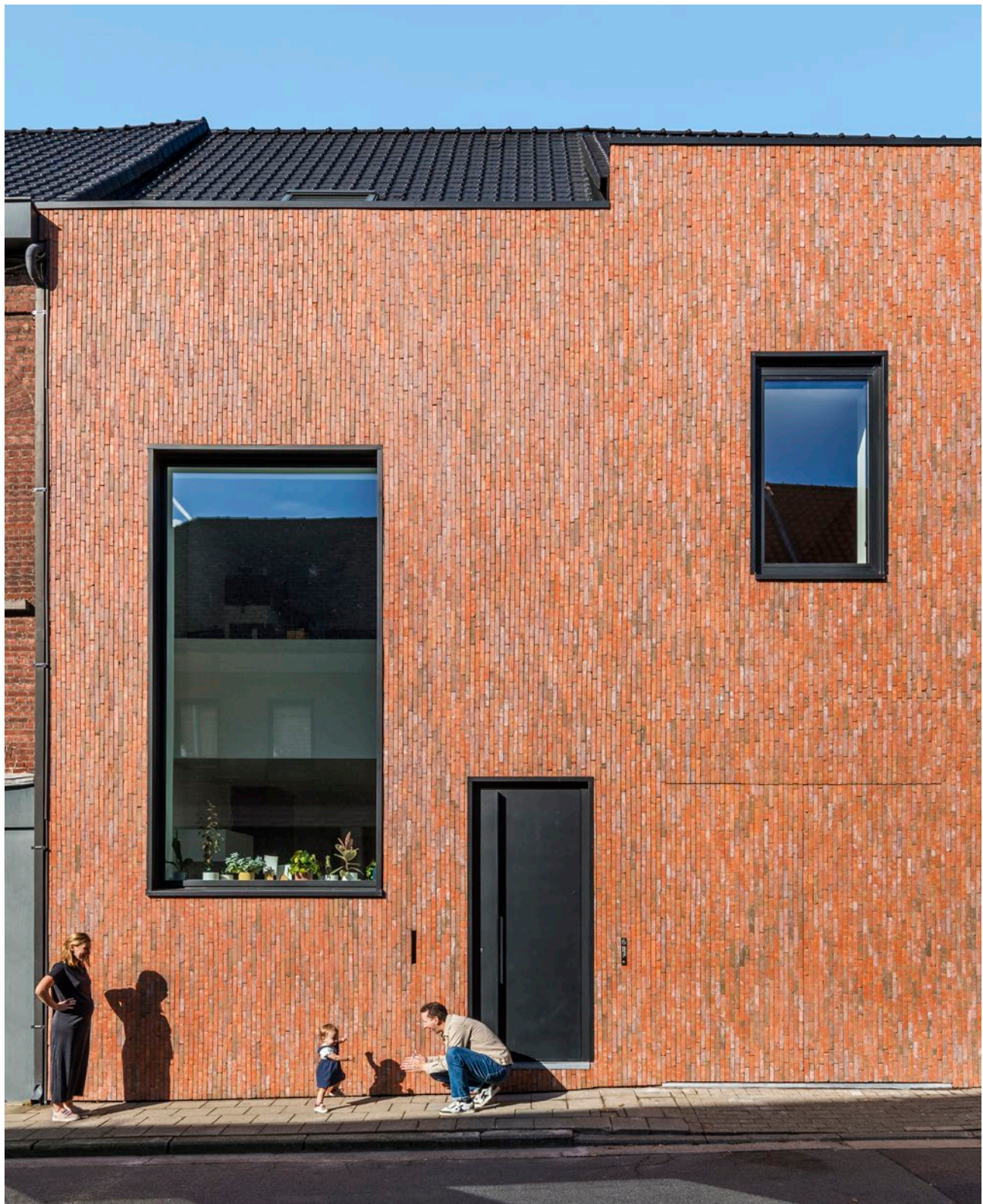
Gevel: Terca Metropolis Aula Rood. Dak: Koramic Stormpan 44 Antraciet.
